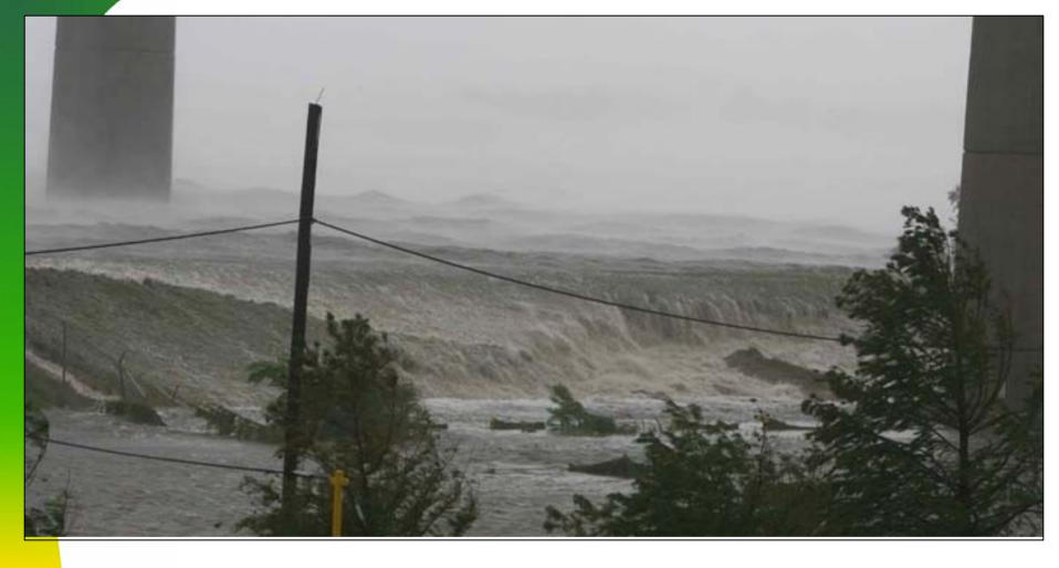
Overtopping: Earthen levee being overtopped at the Entergy Power Plant, Inner Harbor Navigation Channel. This began around 6 AM on August 29<sup>th</sup>. 9 ft storm surge with crest heights up to 17 ft
