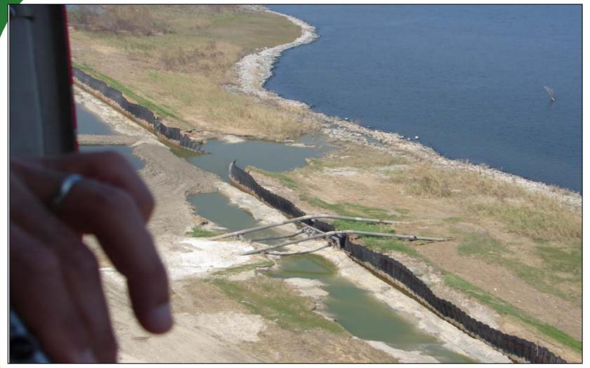
Poor performance: Skeleton of steel sheetpile cutoff walls is all that remains of the MRGO levee between Bayou Bienvenue and Bayou Dupree
