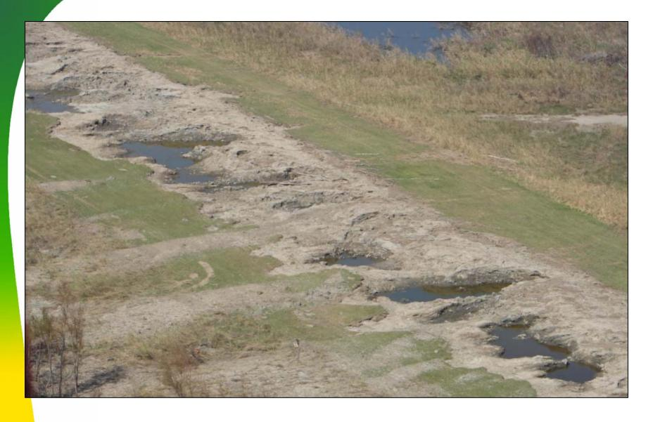
Poor performance: MRGO levee completely washed away about two miles southeast of Bayou Dupree.
