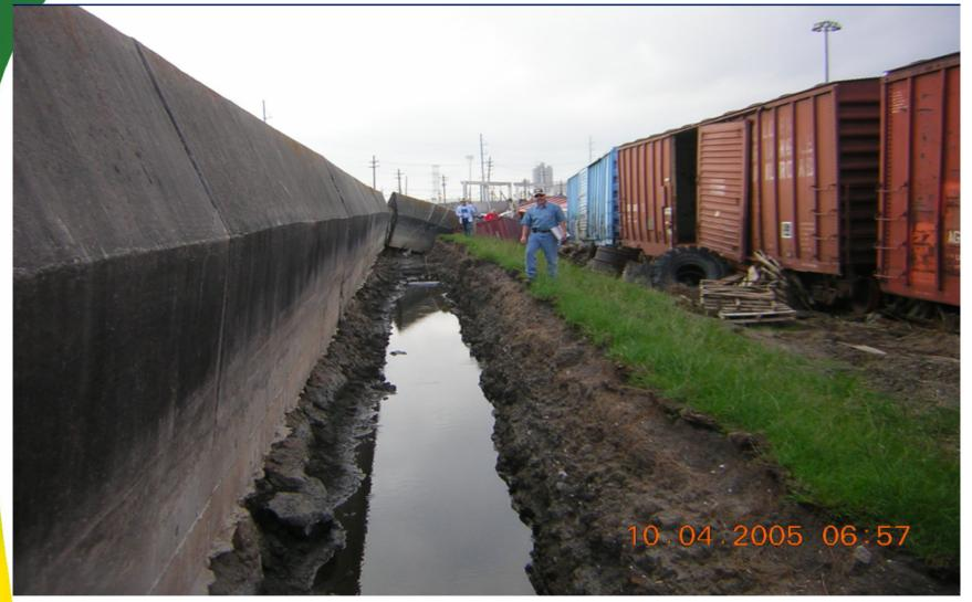
Overtopping scour holes along landside of flood wall on west side of the IHNC. Note broken wall in background. A splash pad on inboard side could have prevented this undercutting for less than 0.5% of the flood wall cost, making the structure "Class 3 survivable."
