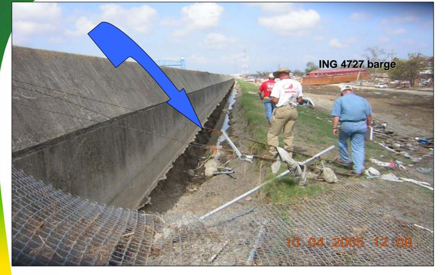
Some sections survived: Evidence of sustained overtopping of concrete flood wall along the IHNC in the Lower Ninth Ward.
